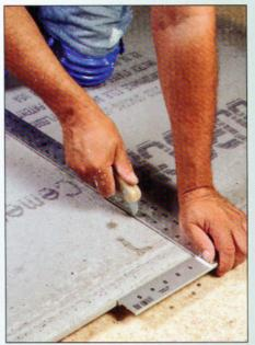
Protect finished floors with a tarp. Backerboard particles will easily scratch a floor. Mark the line to be cut and position a drywall square or metal T square on the line. Using a carbide backerboard scriber and firm pressure, scribe the cut line. Make several passes.
