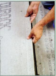
2 While the mortar is still wet, tip the board on a long edge and hinge it toward the floor. Line the first board on a joist and keep a gap of ½ inch between boards, ¼ inch at walls. Manufacturers' directions may vary, but typically you should stagger the joints. Walk on the board to set it in the mortar.
