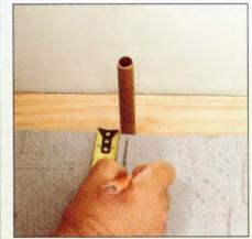
**1** Set the board against the pipe or other obstruction. Mark the diameter of the hole to be cut. Use a tape measure to locate the center of the hole. For faucets measure the location of each faucet hole from the wall and from the tub or floor.
