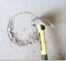
2 Support the cutout with the palm of one hand, if necessary, and tap the scored edge with a hammer. Continue tapping until the surface around the circumference crumbles. Alternatively, drill a series of small holes around the circumference.
