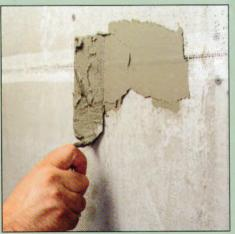
**3** Apply a thin coat of thinset mortar to the taped joint with a margin trowel. Trowel on enough mortar to fill the joint and level it with the backerboard. Feather the edges until they are smooth.
