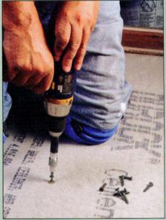
**3** Using a cordless drill and phillips bit, drive backerboard screws through the board and into the subfloor at about 8-inch intervals. Use 2-inch backerboard screws at the joists and 1¼-inch screws in the field. Set the screws so they are flush with the surface of the board.
