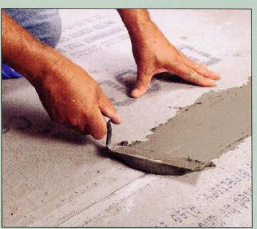
**5** Whether you have used ungummed or pregummed tape, finish the joint by applying a thin coat of thinset mortar over the tape. Use a margin trowel to scoop mortar from the bucket. Apply the mortar so it levels the recess in the joint from side to side. Feather the edges to avoid creating high spots under the tiled surface.
