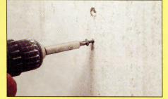
Backerboard fasteners, unlike drywall screws, are made to withstand the rigors of tile installations. Occasionally, however, one will snap off. Check the torque setting of your cordless drill to make sure the clutch slips when the screw just dimples the board. If a backerboard screw snaps, remove the loose piece and drive another about 1 inch away from the first one.
