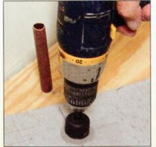
**2** Use a cordless drill and carbide-tipped hole saw or coring saw to cut small holes in backerboard. Place the drill point of the saw on the mark you made, and use light pressure and high speed to cut through the backerboard.
