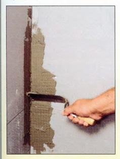
Tape corners with either 2-inch or 4-inch gummed fiberglass mesh tape. In either case do not precut the tape to length. Unroll it as you press it into the joint and cut it when you reach the end. Precut lengths of gummed tape may roll up and stick to themselves before you get them on the board.
