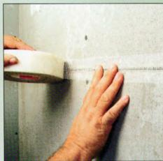
**2** Use 2- or 4-inch gummed tape over each backerboard joint. Press the tape into the joint and unroll it as you go. Use a utility knife to cut the tape at the end of the joint.
