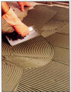
**1** Mix and pour thinset (*page 121*). Hold the smooth side of a notched trowel at a 30-degree angle and spread the mortar in a thick, even coat, forcing it into the subfloor. Then, keeping the notched side of the trowel in contact with the floor and at a 45- to 75-degree angle, work the mortar into ridges.
