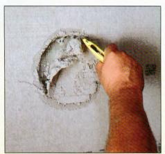
**3** Using a utility knife, cut through the mesh on the opposite side of the board. Push the cutout through and smooth the edges with a rasp, serrated contour plane, or masonry stone.
