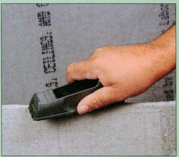
**4** Backerboard cuts are rough, whether made with a carbide scriber or a utility knife. Pieces being joined should have as smooth an edge as possible. Use a contour plane with a serrated blade, a rasp, or a masonry stone to smooth out the edge. Keep the tool perpendicular to the edge of the board and pass over the board several times until its surface is flat.
