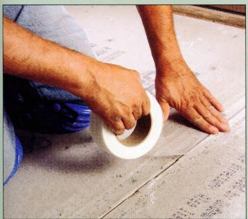
4 Apply 2-inch pregummed fiberglass mesh tape over each joint, pressing the tape firmly on the backerboard. The tape cuts easily with a utility knife. Use 4-inch tape (if available) for increased strength. Alternatively you can embed ungummed tape in a thin coat of mortar applied to the joints. Use this method where stronger joints are required—in stone-tile installations, for example.
