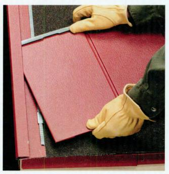
6 Cut a 2" notch for a weep hole in the lip at the bottom left corner of the first shingle. Place the shingle in the bottom left corner of the roof. Interlock the outside edge with the gable trim, and tightly lock the bottom lip to the starter flashing. Fasten to the decking with a minimum of three clips.
