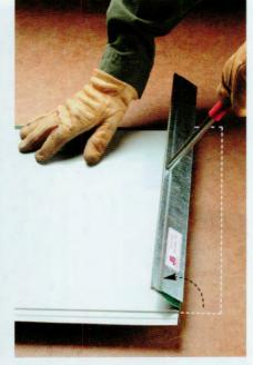
**5** Cut a 1½" notch in the end of the ribs of the first roofing panel. Bend the flat part of the panel back 180° to create a hem, using a hemming tool. Apply sealant in the panel hem.
