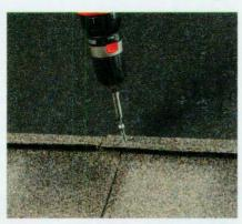
3 Drive a number 8 hex head, corrosion-resistant screw through the upper left corner of the shingle. Drive a screw in the top right-hand corner, and two screws in between the corners.
