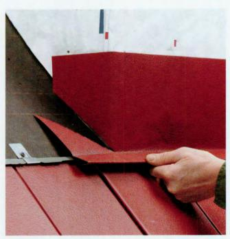
**10** If your roof has a dormer, install shingles as close to the front of the dormer as possible. Cut and bend trim coil to fit under the siding or flashing and overlap the last row of shingles. Nail the flashing to the dormer and caulk the nail heads.
