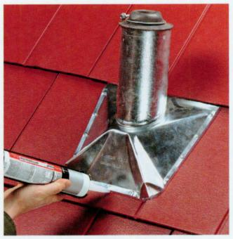
**12** Cut shingles to fit snugly around pipes. Install a panel over the pipe, folding back the top locking edge on the shingle above the pipe where the flashing will sit. Place the pipe flashing over the pipe and fasten with screws that are long enough to penetrate the roof decking. Caulk around the flashing. Set the next row of shingles over the flashing.
