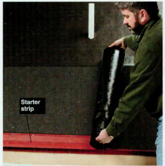
**1** Cover the roof with ice guard and felt paper (pages 62 to 63), then place the starter flashing tight against the fascia. Nail the starter strip to the roof deck and fascia every 18". Overlap starter strips by 2" if more than one is needed. Place a layer of ice and water shield over the starter strip.
