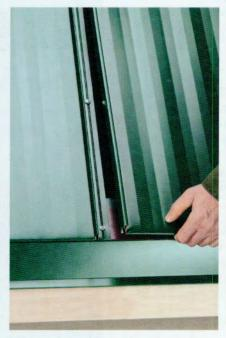
7 Notch and hem the second panel, following step 5. Apply sealant in the hem. Snap the second panel over the first and place against the offset cleat. Fasten in place with screws. Install remaining panels the same way.
