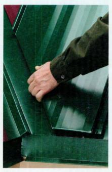
8 Cut panels parallel to the valley, using aviation snips. Notch and hem panels to fit the offset cleats along the valley, using the hemming tool. Fill the hem with a bead of sealant, then install over the offset cleat.
