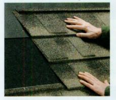
**1** Following the manufacturer's recommended offset, install the shingles one row at a time. Overlap shingles so the top panel clicks into the lock of the underlying panel.
