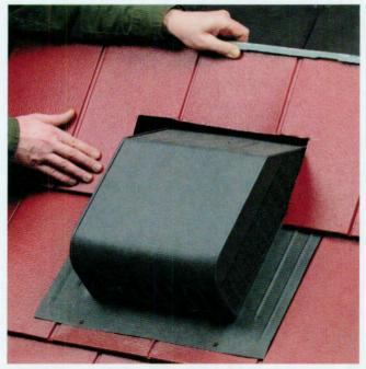
**13** Cut shingles to match the roof holes for each louver. Install the shingles over the holes. Fold back the top lock on the shingle where the louver will sit. Install the roof louver over the shingles, fasten with screws that penetrate the roof decking, and caulk around the louver flashing. Place the next row of shingles over the back edge of the louver flashing.
