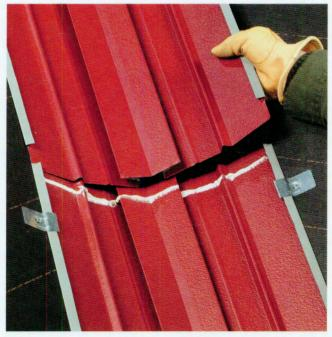
**5** To overlap valley pans, cut the locking lips  $1\frac{1}{2}$ " from the bottom edge on the overlapping piece. Apply sealant to the end of the first valley pan, then overlap it  $1\frac{1}{2}$ " with the second piece. Fasten a clip over both valley pans at the seam.
