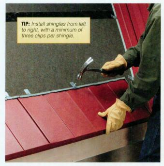
7 Cut a 2" weep hole in the second shingle and set it in place so it interlocks with both the first shingle and the starter flashing. Fasten with clips. Install the remaining shingles in the first course the same way, interlocking the edges. Note: Remaining courses of shingles do not have weep holes.
