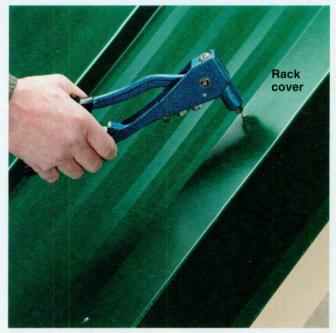
**9** Place tape sealant next to the rib along the rake end. Set a z-closure over the tape and install with wood screws every 12". Place tape sealant over the top leg of the z-closure. Fasten a cleat to the rake of the house at a height that allows the rake cover to fit over the cleat and lie flat over the z-closure. Slide the rack cover over the cleat and fasten to the z-closure, using a rivet gun with pop rivets every 12".
