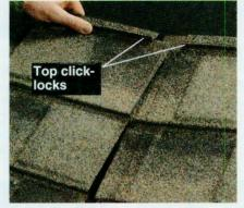
2 Keep the top edges of adjacent panels flush. Slide panels together so the gap between the top clip-locks is no more than  $\frac{3}{6}$ ".
