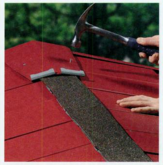
**14** Cut shingles flush with hips and ridges. Cut 4"wide strips of ice guard and place them over hips and ridges. Set the first ridge cap over the ice guard at one end of the roof, overlapping the gable flashing. Face nail the ridge cap in place, then caulk the nail heads.
