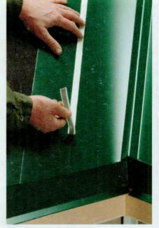
**3** Center the valley flashing over the valley and tack it in place with screws every 48". Fasten tape sealant along both sides of the valley, 5" from the center.
