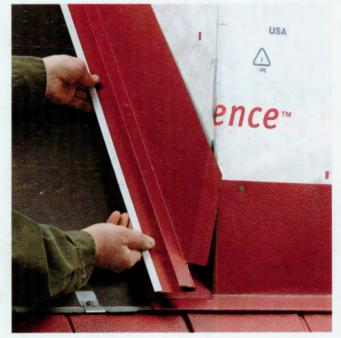
**11** To complete the dormer, place the sidewall flashing against the dormer, overlapping the trim coil installed in step 10. If the dormer is sided, slide the flashing under the siding. Nail to the dormer. Cut shingles to fit in the sidewall flashing.
