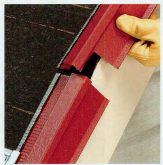
**3** Where more than one gable trim flashing is needed, cut 1½" notch from the bottom of the channel of the overlapping piece, then overlap the trim flashings 1½".
