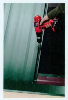
6 Set the panel over the offset cleat, starting at the rake edge. Square the panel to the eave flashing. Drive truss head screws in the center of the fastening groove on the panel's male (right) side.
