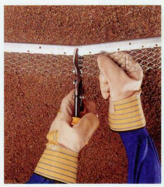
**Use aviation snips** to trim the excess lath, edging, and drip screed. Wear safety goggles and heavy gloves as protection from sharp edges.
