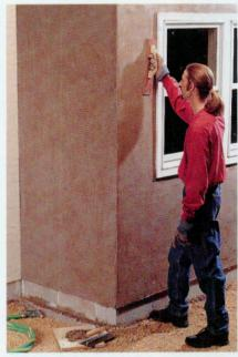
4 Mist the surface occasionally for 48 hours. Mix and apply the brown coat approximately %" thick, then level the entire surface with a wood darby to provide a roughened gripping surface for the finish coat.
