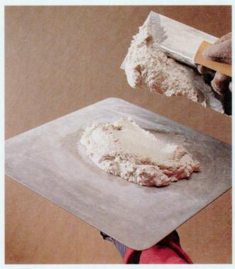
**Mix the finish batch** so it contains slightly more water than the scratch and brown soats. The mix should still stay on the mortar hawk without running.
