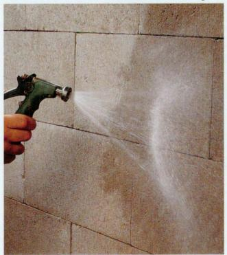
$\blacksquare$  Starting near the top of the wall, mist a 2 × 5-ft. section on one side of the wall with water to prevent the blocks from absorbing moisture from the cement once the coating is applied.
