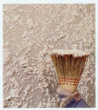
**Achieve a wet-dash finish** by flinging, or dashing, stucco onto the surface. Let the stucco cure undisturbed.
