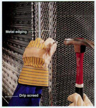
**Install metal edging** along edges of walls, and drip screed (also called weep screed) at the base to achieve clean corners and edges. Make sure edging is level and plumb, then attach it with roofing nails.
