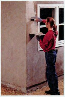
**5** Mix the finish coat, adding tint as required, and slightly more water than in previous coats. The mix should still sit on the mortar hawk without running. Apply the finish coat so the edging is fully embedded (about 1/6" thick).
