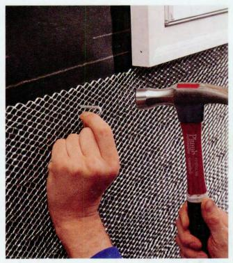
Install self-furring expanded metal lath over the building paper with 1½" roofing nails driven into studs every 6". Sheets of lath should overlap 1" horizontally and 2" vertically. Make sure the lath is installed with the rougher side facing out.
