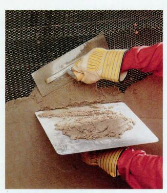
Begin at the top or the bottom of the wall. Hold a mortar hawk close to the wall, and press stucco into the lath with a square-end trowel. Press firmly to fill voids, and cover the mesh as smoothly as possible.
