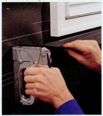
Attach building paper to wood frame construction, using heavy-duty staples or roofing nails. Overlap seams by 4". In some regions, more than one layer of building paper may be required. Ask your local building inspector about code specifications.
