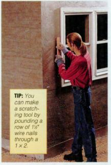
Wait for the scratch coat to harden enough so an impression remains when you press on it. Rough up the surface by making shallow horizontal scratches the length of the wall.
