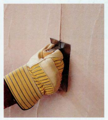
4 To prevent random cracking, use a groover to cut control joints from the top to the bottom of the wall, every 4 ft. for a 2-ft.-high wall, and every 8 ft. for a 4-ft.-high wall. Seal hardened joints with silicone caulk.
