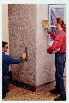
**5** Finish the surface by throwing stucco at the wall with a whisk broom, then flattening the stucco with a trowel. Wait 24 hours for the finish coat to set up, then mist 2 to 3 times a day for two days, and once a day for another three days.
