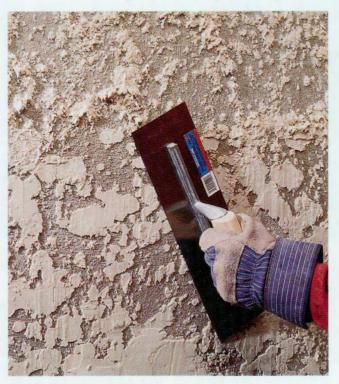
For a dash-trowel texture, dash the surface with stucco, using a whisk broom (left), then flatten the stucco by troweling over it.
