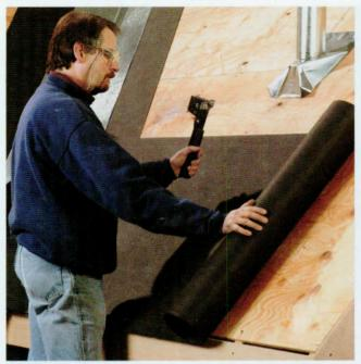
Prepare the roof decking by installing valley flashing at all valleys (pages 66 to 67). Apply felt paper underlayment to the first 36" of the roof deck. Note: Depending on your climate and building codes, you may want to install ice and water shield for this step rather than felt paper.
