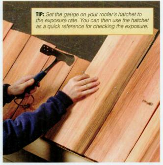
**3** Set the first course of shakes over the starter row, aligning the shakes along the rake ends and bottoms. Joints between shakes must overlap by at least 1½". Drive two nails in each shake, ¾" to 1" from the edges, and 1½" to 2" above the exposure line. Use the hatchet to rip shakes to fit.
