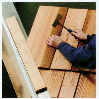
**6** Use the  $1 \times 4$  to align the edge of the shakes along the valley. Keep the  $1 \times 4$  butted against the valley center, and place the edge of the shake along the edge of the board. Avoid nailing through the valley flashing when installing the shakes.
