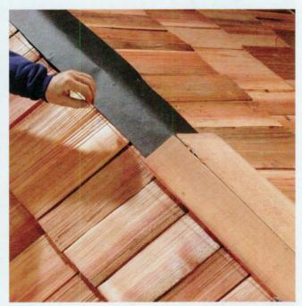
14 Cut 8" strips of felt paper and staple them over the hips and ridge. Set a factory-made hip and ridge cap at one end of the ridge, aligned with the roof peak. Do the same at the other end of the roof. Snap a chalk line between the outside edges of the caps.
