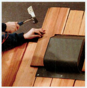
11 Apply roofing cement along the underside of the roof louver flange, then set it over the vent cutout and over the shakes directly below it. Nail the louver in place. Install shakes over the sides and back of the louver, trimming to fit, as needed.
