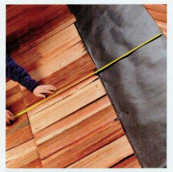
12 As you approach the ridge, measure from the last installed row to the peak. Do this on each side of the roof. If the measurements are not equal, slightly adjust the exposure rate in successive rows until the measurements are the same. Make sure you're measuring to points that are aligned at the peak. The top of the sheathing is probably not level across the roof and cannot be a reference point.
