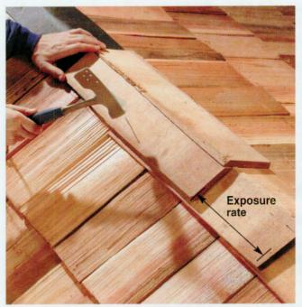
15 Set a ridge cap along the chalk line, flush with the edge of the roof, to serve as the starter. Install with two nails. Place a cap directly on top of the starter cap, and nail in place. Install caps along the remainder of the ridge, alternating the overlap pattern. The exposure rate should be the same as the roof shakes. Nails should penetrate the roof decking by ½".
