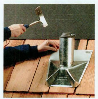
**7** Notch shakes to fit around a plumbing stack, using a jig saw, then install a course of shakes below the stack. Apply roofing cement to the underside of the stack flashing, then place it over the stack and over the shakes. Nail the flashing along the edges.
