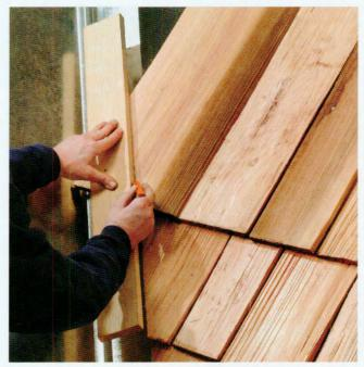
$\bf 5$  Set shakes in place along valleys, but don't nail them. Hold a 1  $\times$  4 against the center of the valley flashing without nailing it. Place it over the shakes to use as a guide for marking the angle of the valley. Cut the shakes, using a circular saw, then install.
