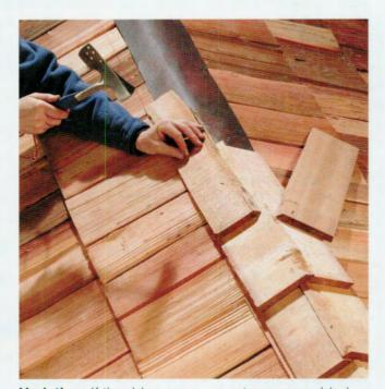
**Variation:** If the ridge caps are not pre-assembled by the manufacturer, install the first cap along the chalk line, then place the second cap over the edge of the first. Alternate the overlap pattern across the ridge.
