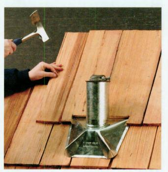
Overlap the exposed flashing with the next row of shakes. Cut notches in the shakes to fit around the stack, keeping a 1" gap between the stack and shakes.
