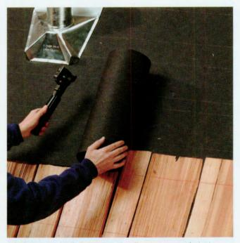
A Snap a chalk line over the first course of shakes at the exposure line. Snap a second line at a distance that's twice the exposure rate. Staple an 18"-wide strip of felt paper at the second line. Overlap felt paper vertical seams by 4". Install the second course of shakes at the exposure line, offsetting joints by 1½" minimum. Install remaining courses the same way.
