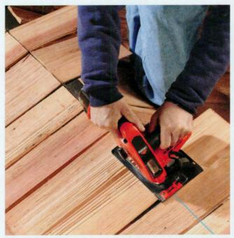
13 Run shakes past the roof peak. Snap a chalk line across the shakes at the ridge. Set the circular saw blade to the depth of the shakes, then cut along the chalk line.
