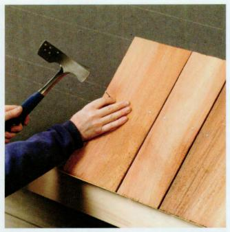
2 Install a starter shake so it overhangs the eaves and rake edge by 1½". Do the same on the opposite side of the roof. Run a taut string between the bottom edges of the two shakes. Install the remaining shakes in the starter row, aligning the bottoms with the string. Keep the manufacturer's recommended distance between shakes, usually ¾" to ¾".
