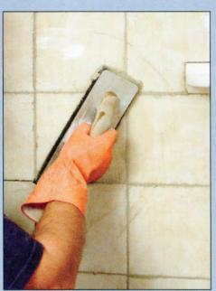
When the adhesive is dry, clean the J surface and joints of any remaining excess. Mix grout and apply it with a grout float, forcing it into the joints in both planes. Let the grout cure until a damp sponge won't lift the grout out of the joints.
