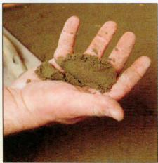
The mortar for a shower enclosure should be just wet enough to clump together. You'll know it's right when you squeeze it and it just holds its shape.
