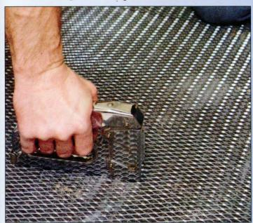
Cut a piece of 15-pound felt to fit the floor area between the bottom plates or the \(^34\)-inch float guides and staple the felt to the floor. Cut a section of metal lath to the same dimensions. The metal gives the floor a "tooth" for the mortar. Set the metal lath in place and snip out a circle about an inch wider than the circumference of the drain. Staple the entire sheet of metal lath securely to the floor, flattening any bumps which could weaken the sub-base.
