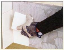
Tile the bench as you would a wall, lining up the courses on the front of the bench with the courses on the walls. Finish tiling the shower and grout the entire installation. Seal the grout with the product recommended by the manufacturer.
