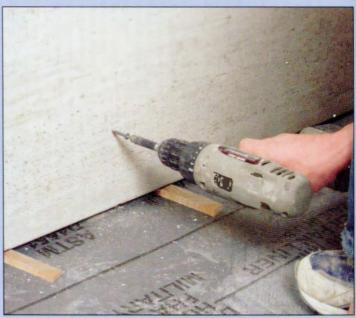
2 Clean off any grit with a damp cloth. As added protection you can cover the liner with a drop cloth to prevent a backerboard corner from puncturing it. Cut backerboard to fit the walls and set it on ½-inch shims. Fasten the backerboard to the studs with backerboard screws (page 94); keep the screws within the top 1 inch of the pan membrane. Remove the shims and caulk the space at the bottom with silicone. Tape and mud the seams with modified thinset.
