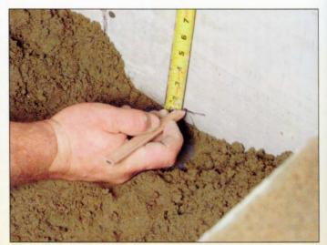
**2** The floor of the pan must slope ½ inch for every linear foot. Compute the amount of slope based on the dimensions of the enclosure and mark this point on the backerboard.
