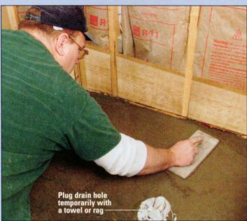
Using bagged sand mix from your home center (or 4 parts sand, 1 part portland cement), mix up a batch of dry deck mud with latex additive (not water). Mix the mortar in a wheelbarrow (not a bucket). Dump the mortar onto the floor, spreading it with a wood float and sloping it from the top of the guides (or the bottom wall plate on larger stalls) to the top of the drain flange. Compact the mortar into an even surface and let it dry overnight.
