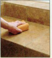
When the mortar has cured, grout the joints and clean the tile. When the grout has cured, seal the grout lines.
