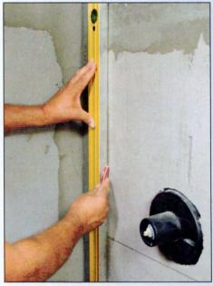
Using a dimensional layout drawing, locate the point on which a horizontal and vertical grout line will fall. Hold a 4-foot level on both planes and mark reference lines. Then snap layout grids whose dimensions equal the width of the tiles and grout joints.
