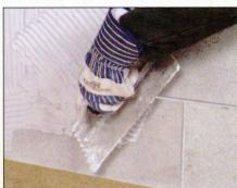
Spread mortar on the shower pan and set concrete block in the mortar. Plumb and level the block. Mortar the side pieces in place and repeat the process for the next course(s) of block. Then spread a level coat of thinset on the surfaces to be tiled.
