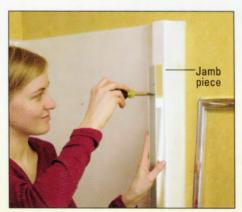
Measure the opening and select a door with a frame you can adjust to fit your unit. Follow manufacturer's instructions. In general you'll begin by cutting the jamb piece to size and installing a bottom track and seal. Each jamb is made of two interlocking pieces. One attaches
