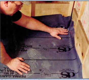
Set the membrane on the floor of the enclosure and unroll it from I front to back, pulling it forward until it covers the front of the curb. Working from the drain outward, smooth out the air bubbles. Then staple the top 1 inch of the sheet to the blocking. Weld the corners and cut the sheet at the bottom of the jambs. Fold the sheet over the curb and tack it only on the front. Solvent-weld a dam corner (available from the manufacturer) over the jamb cuts.
