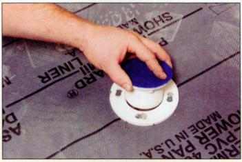
Wrap the threads of the strainer with four or five turns of plumber's tape and screw the strainer into the flange. To protect the strainer and drain from stray mortar and thinset, apply two layers of crisscrossed masking tape. Overlap the tape and cut it flush around the edge of the strainer.
