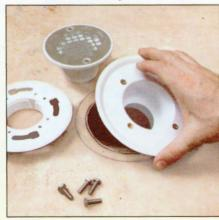
Cut a hole in the floor with a hole saw or iigsaw (drilling a starter hole first). Coat the bottom of the lower drain with beads of silicone—one outside and one inside the bolt circle.
