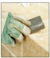
Cover all the framing with a waterproof membrane and backerboard. Caulk all seams with silicone. Tile the seat surfaces first, followed by the wall tile. Use bullnose for the edges or round the field tile with a masonry stone.
