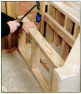
Make sure your plan for a bench includes exact dimensions. Measure each framing member before cutting and fastening it. Mistakes in shower stalls are certain to leak. Frame the rear wall of the bench first, then each front wall.
