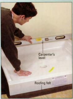
**2** Place a layer or two of roofing felt to smooth any unevenness in the floor. (Some manufacturers may require a bed of mortar or sand.) Set the shower base over the drain to confirm that the drain is positioned where you want it. Check for level; shim with roofing felt as needed.
