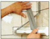
When you set the wall surface, leave a space for surfacemounted accessories, such as soap dishes, cutting the tile around it if necessary. Use a margin trowel to apply mortar to both the recess and the back of the accessory and press the unit into place. Keep it centered with wedges. Tape it in place until the mortar dries, then caulk the joint.
