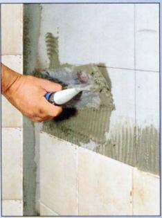
**2** Tack a batten on the bottom of the wall, if necessary (page 124) and prepare enough adhesive to cover the number of layout grids you can lay before the adhesive begins to set up. Set field tiles on the back wall first. Don't set tiles around fixtures yet.
