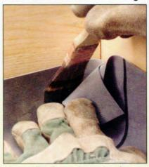
After stapling the membrane along its length, you will have excess material at the corners. Fold the corners into triangles and solvent-weld the folds in place.
