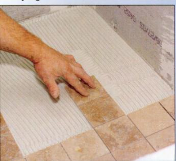
When the floor has dried, scape off any remaining imperfections with a steel trowel, then spread and comb latex-modified thinset. Press the tiles firmly into the mortar to make sure they conform to the slope of the floor. Line up all the edges with a 2-foot straightedge and let the mortar cure overnight. Grout the tiles with latex-modified grout, cleaning off the excess and wiping the grout haze.
