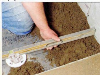
**1** Using a torpedo level or 2-foot level (the longest size that will fit the enclosure), transfer the plane of the bottom of the strainer to the walls and the curb. Mark the plane on the backerboard with a felt-tip pen.
