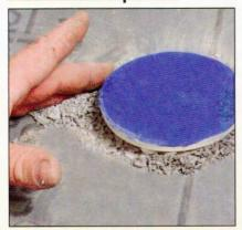
Weep holes allow moisture trapped in the mortar bed to escape down the drain. If the moisture can't go down, it will go up-into your grout, causing mold and mildew. To keep the weep holes from clogging with mortar, put a few spacers or pieces of gravel around them.
