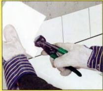
Cut the tile at the corner of the tub carefully. This cut can be somewhat tricky, so it's best to lay out the curve on a cardboard template and transfer the line to the tile. Make relief cuts and bite out the curve with nippers.
