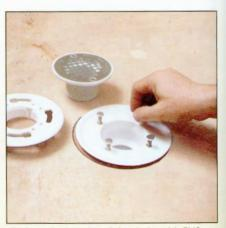
Coat the interior of the drain with PVC primer and cement and twist the drain onto the waste line. Let the cement dry and insert the drain bolts into the lower drain plate, leaving about 3/4-inch exposed.
