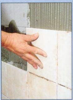
**3** When the back wall is done, set the side walls. Start from the front, leaving cut tiles for the back edge at the corner of the adjoining wall. Tape the tiles if necessary to hold them in place (page 124). Remove excess adhesive from the joints; let it cure.
