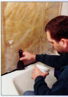
Apply asphalt roofing cement to the flange of the tub. This is the place where most tub and shower surrounds fail, and water that gets into this joint will migrate upwards and down into the floor. The asphalt cement seals the tub to the waterproofing felt or 4-mil poly sheet.
