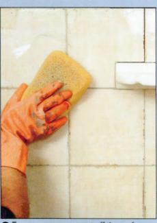
To scrape excess grout off the surface, I hold the float almost perpendicular to the tile and work diagonally to avoid pulling the grout from the joints. Dampen a sponge, wring it out thoroughly, and clean the surface twice, smoothing the joints. Scrub off the haze with a clean rag.
