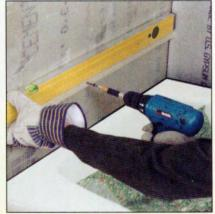
To keep the first row (and all that follow) level, tack a 1x batten to the backerboard one full tile width above the tub. Cover the tub with heavy paper to protect it from damage it might incur as you tile the wall.
