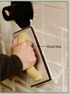
A Mix a batch of latex-reinforced grout and use a grout float to first push the grout into the joints; then scrape away most of the excess. Wipe several times with a damp sponge, working to create consistent grout lines. Allow to dry and buff with a dry towel. Caulk all the inside corners.
