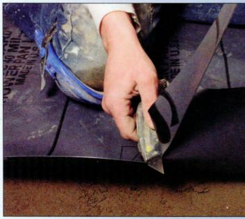
Roll out the membrane on the surrounding floor. Mark the cut lines 9 inches larger than the shower floor on the sides and back, and 16 inches larger in the front (to cover all faces of the curb). If the stall is larger than the membrane, solvent-weld additional sections. Reinforce the drain area by solvent-welding a 10-inch circle of membrane in the center, folding the edges, and rolling or folding the membrane so it fits easily in the enclosure.
