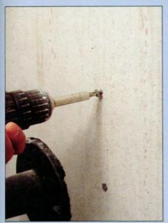
Cut backerboard so its edges will be I centered on the studs and fasten it to the studs with backerboard screws. When fitting backerboard above a tub, leave a 1/4-inch gap between the bottom edge of the board and the tub rim.
