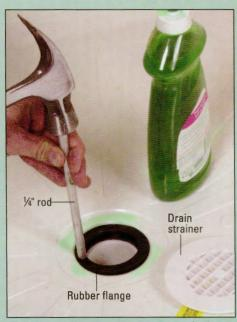
3 Using liquid soap as a lubricant, fit the rubber flange (provided with the shower base) over the drain extension and push it as far down as you can. Tap it all the way in place with a 1/4-inch steel rod. Install the drain strainer.
