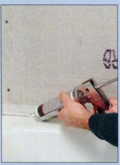
Caulk the gap at the bottom of the J backerboard with clear or white silicone caulk. The caulk seals the joint between the tub and backerboard and allows for some expansion and contraction of the different materials.
