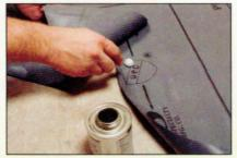
If the shower enclosure is larger than the CPE or PVC sheet, you will need to seam an additional section. Coat both sides of the seam with the primer or sealer appropriate to the material, covering about 4 inches from the edges. Let the primer dry. Overlap the edges and roll them tightly. After 5 minutes, try to separate the seam. If it comes apart, repeat the process.
