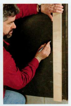
Place the story pole at a corner, aligning the bottom with the chalk line. Transfer the marks onto the wall. Do this at each corner, door, and window location.
