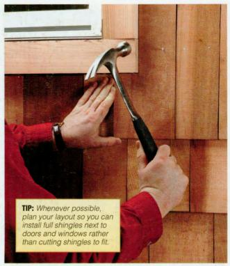
10 Cut shingles to fit around doors, windows, and protrusions in the walls, using a coping saw or handsaw. Make sure gaps between shingles aren't aligned with the edges of doors and windows.
