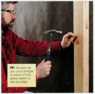
**5** Place a  $1 \times 3$  board at an outside corner, aligning it with the chalk line at the bottom. Keep the outside edge flush with the adjacent wall. Nail it in place. Overlap the edge of the board with a  $1 \times 4$ , align it with the chalk line, and nail in place. If more than one trim board is needed to span the length of the wall, miter the ends at  $45^{\circ}$  and place them together. Do this for all outside corners.
