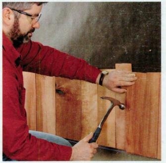
Place the first course of shingles over the starter row, flush with the chalk line at the bottom. Overlap the seams in the starter course by at least 1½".
