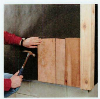
**7** If the chalk line is hard to see, run a string from the bottom of the corner trim pieces. Starting at a corner, install the starter row of shingles, ½" above the chalk line. Keep the manufacturer's recommended distance between shingles and between shingles and trim, usually a ½" to ½" gap. Keep nails ¾" from edges and 1" above the line of exposure.
