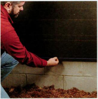
2 Starting at the lowest corner of the house, snap a level chalk line at the bottom of each wall where the siding will start. Measure the height of the wall from the chalk line to the soffits.
