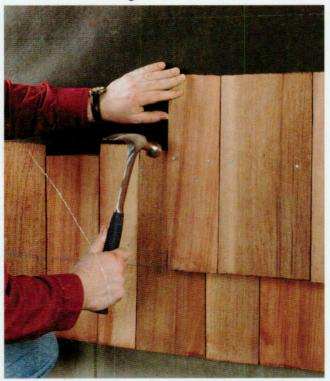
9 Snap a chalk line across the shingles to mark the exposure, using the reference lines from step 4. Install a course of shingles at the chalk line, offsetting the seams. Install remaining rows the same way.
