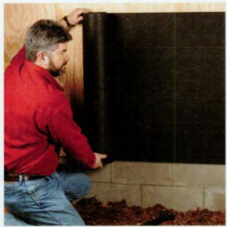
Cover the exterior sheathing with felt paper. Starting at the bottom of a wall, install the paper horizontally, using staples. Wrap corners a minimum of 4". Overlap vertical seams 6" and horizontal seams 2". Cut out openings around doors and windows.
