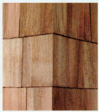
**Mitered corners** are made by cutting corner shingles at a 45° angle and butting them together. This method is very time consuming.
