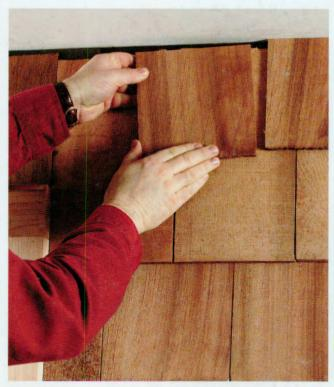
13 Measure and cut the last row of shingles to fit under the horizontal eaves. Leave the recommended gap between shingles and soffits. Nail the shingles in place.
