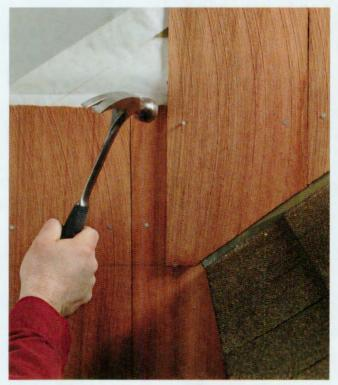
**12** When applying shingles on a dormer or above a roof line, keep the bottom edge of the shingles ½" above the roof shingles. Cut shingles with a handsaw or circular saw.
