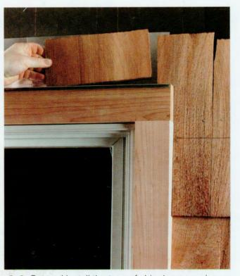
11 Cut and install the tops of shingles over windows and doors. Align the tops with adjacent shingles on either side of the door or window.
