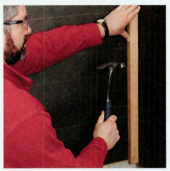
**6** Fasten a  $2 \times 2$  in an inside corner, flush with the chalk line at the bottom. If more than one board is needed to span the height of the wall, miter the adjoining ends at  $45^{\circ}$  and butt them together.
