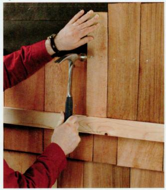
**Option:** To ensure straight lines, tack a 1 × 4 flush with your reference lines. Nail the board through gaps between shingles. Use the board as a guide for installing the shingles.
