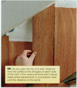
14 Use a T-bevel to determine the roof angle on the gable end of the house. Cut shingles at this angle for each row at the gable end, using a handsaw or circular saw. Install shingles up to the peak.
