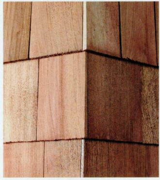
**Woven corners** have shingles that overlap at the corners for a weave effect. This overlap alternates between walls with each successive course.
