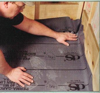
Set the membrane on the floor of the enclosure and unroll it from front to back, pulling it forward until it covers the front of the curb. Working from the drain outward, smooth out the air bubbles. Then staple the top 1 inch of the sheet to the blocking. Weld the corners and cut the sheet at the bottom of the jambs. Fold the sheet over the curb and tack it only on the front. Solvent-weld a dam corner (available from the manufacturer) over the jamb cuts.
