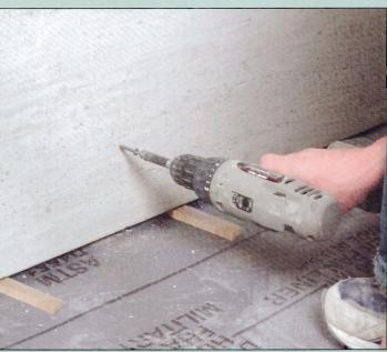
2 Clean off any grit with a damp cloth. As added protection you can cover the liner with a drop cloth to prevent a backerboard corner from puncturing it. Cut backerboard to fit the walls and set it on ½-inch shims. Fasten the backerboard to the studs with backerboard screws (page 194); keep the screws within the top 1 inch of the pan membrane. Remove the shims and caulk the space at the bottom with silicone. Tape and mud the seams with modified thinset.
