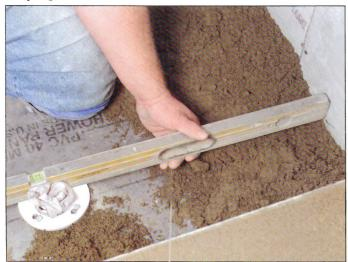
Using a torpedo level or 2-foot level (the longest size that will fit the enclosure), transfer the plane of the bottom of the strainer to the walls and the curb. Mark the plane on the backerboard with a felt-tip pen.
