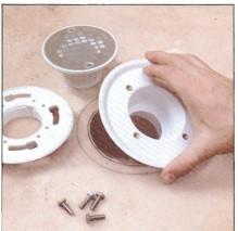
Cut a hole in the floor with a hole saw or jigsaw (drilling a starter hole first). Coat the bottom of the lower drain with beads of silicone—one outside and one inside the bolt circle
