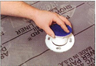
Wrap the threads of the strainer with four or five turns of plumber's tape and screw the strainer into the flange. To protect the strainer and drain from stray mortar and thinset, apply two layers of crisscrossed masking tape. Overlap the tape and cut it flush around the edge of the strainer.
