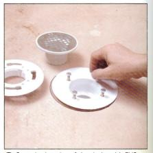
Coat the interior of the drain with PVC primer and cement, and twist the drain onto the waste line. Let the cement dry, then insert the drain bolts into the lower drain plate, leaving about \(^{3}\)4 inch exposed.
