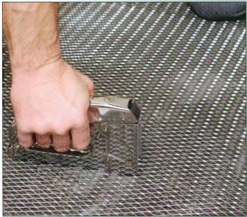
Cut a piece of 15-pound felt to fit the floor area between the bottom plates or the ¾-inch float guides, and staple the felt to the floor. Cut a section of metal lath to the same dimensions. The metal gives the floor a "tooth" for the mortar. Set the metal lath in place and snip out a circle about an inch wider than the circumference of the drain. Staple the entire sheet of metal lath securely to the floor, flattening any bumps that could weaken the subbase.
