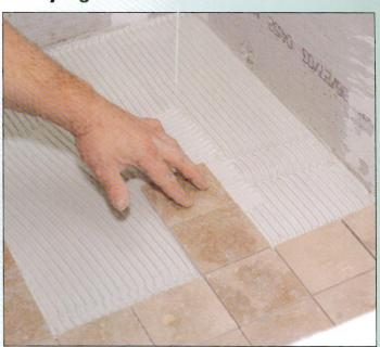
When the floor has dried, scrape off any remaining imperfections with a steel trowel, then spread and comb latex-modified thinset. Press the tiles firmly into the mortar to make sure they conform to the slope of the floor. Line up all the edges with a 2-foot straightedge and let the mortar cure overnight. Grout the tiles with latex-modified grout, cleaning off the excess and wiping off the grout haze.
