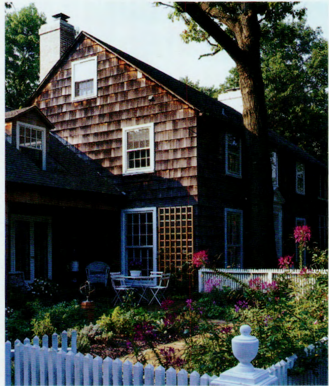
Shakes and shingles closely resemble each other, although shingles are thinner and smaller than shakes. Most authentic shakes and shingles are made of Western cedar.
