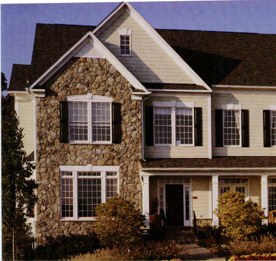
Combining two types of siding can enhance the curb appeal of your home. This house features stone and fiber cement siding.
