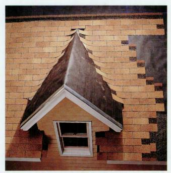
**9** Shingle upward from the eaves on the unshingled side of the obstruction, using the vertical line as a reference for re-establishing your shingle slot offset pattern. Fill out the shingle courses past the rake edges of the roof, then trim off the excess.
