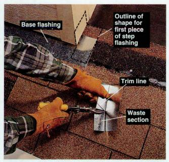
Shingle up to an element that requires flashing, so the top of the reveal areas are within 5" of the element. Install base flashing, using the old base flashing as a template. Bend a piece of step flashing in half and set it next to the lowest corner of the element. Mark a trim line on the flashing, following the vertical edge of the element. Cut the flashing to fit.
