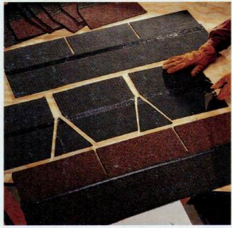
**23** Cut three 12"-square cap shingles from each 3-tab shingle. With the back surface facing up, cut the shingles at the tab lines. Trim the top corners of each square with an angled cut, starting just below the seal strip to avoid overlaps in the reveal area.
