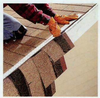
Mark and trim the shingles at the rake edges of the roof. Snap a chalk line %" from the edge to make an overhang, then trim the shingles.
