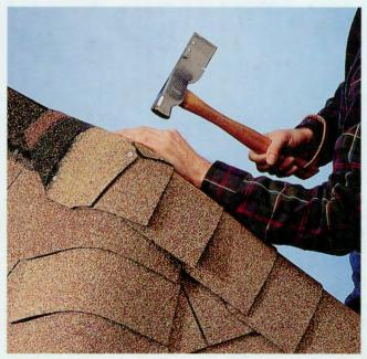
Shingle the hips in the same manner, using a chalk reference line and cap shingles. Start at the bottom of each hip and work to the peak. Where hips join with roof ridges, install a custom shingle cut from the center of a cap shingle. Set the cap at the end of the ridge, and bend the corners so they fit over the hips. Secure each corner with a roofing nail, and cover the nail heads with roofing cement.
