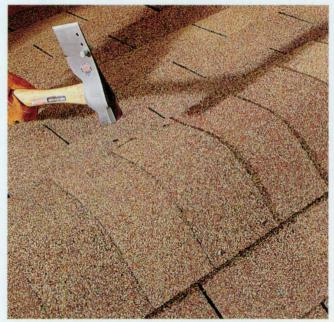
Following the chalk line, install cap shingles halfway along the ridge, creating a 5" reveal for each cap. Then, starting at the opposite end, install caps over the other half of the ridge to meet the first run in the center. Cut a 5"-wide section from the reveal area of a shingle tab, and use it as a "closure cap" to cover the joint where the caps meet.
