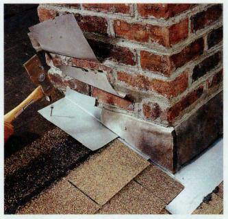
Install step flashing and shingles, working up to the high side of the chimney. Fasten flashing to the chimney with roofing cement. Fold down the counterflashing as you go.
