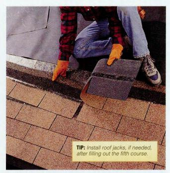
**6** Fill in shingles in the second through fifth courses, working upward from the second course and maintaining a consistent 5" reveal. Slide lower-course shingles under any upper-course shingles left partially nailed, and then nail them down.
