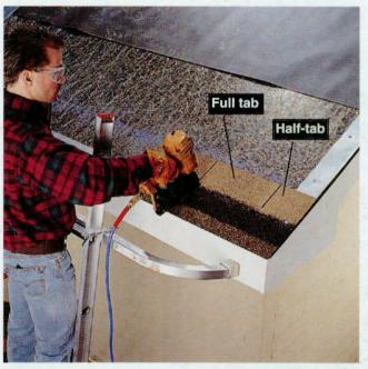
2 Trim off one-half (6") of an end tab on a shingle. Position the shingle upside down, so the tabs are aligned with the chalk line and the half-tab is flush against the rake edge. Drive %" roofing nails near each end, 1" down from each slot, between tabs. Butt a full, upside-down shingle next to the trimmed shingle, and nail it. Fill out the row, trimming the last shingle flush with the opposite rake edge.
