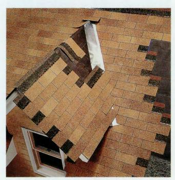
**11** Install shingles on adjoining roof decks, starting at the bottom edge, using the same offset alignment pattern shown in steps 1 to 6. Install shingles until courses overlap the center of the valley flashing. Trim shingles at both sides of the valley when finished.
