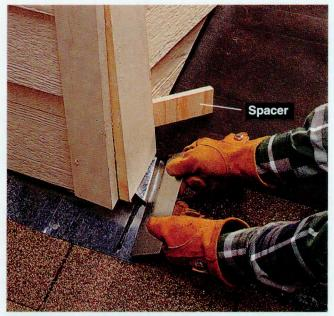
Pry out the lowest courses of siding and any trim at the base of the element. Insert spacers to prop the trim or siding away from the work area. Apply roofing cement to the base flashing in the area where the overlap with the step flashing will be formed. Tuck the trimmed piece of step flashing under the propped area, and secure the flashing. Fasten the flashing with one rubber-gasket nail driven near the top, and into the roof deck.
