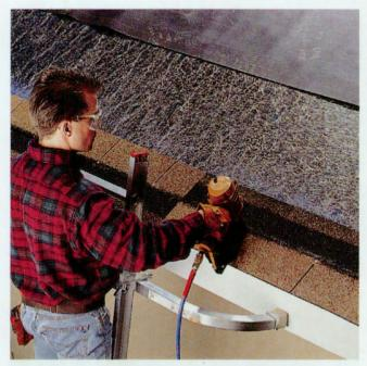
3 Apply the first full course of shingles over the starter course, with the tabs pointing down. Begin at the rake edge where you began the starter row. Place the first shingle so it overhangs the rake edge by %" and the eaves edge by ½". Make sure the top of each shingle is flush with the top of the starter course, following the chalk line.
