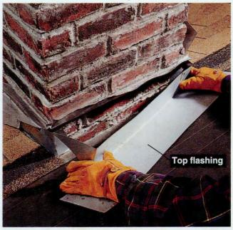
**21** Cut and install top flashing (also called a saddle) around the high side of the chimney. Overlap the final piece of flashing along each side. Attach the flashing with roofing cement applied to the deck and chimney, and with rubber-gasket nails driven through the flashing base into the roof deck. Shingle past the chimney, using roofing cement (not nails) to attach shingles over the flashing.
