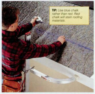
**1** Cover the roof with felt paper (pages 62 to 63) and install drip edge (pages 64 to 65). Snap a chalk line onto the felt paper or ice guard, 11½" up from the eaves edge, to mark the alignment of the starter course. This will result in a ½" shingle overhang for standard 12" shingles.
