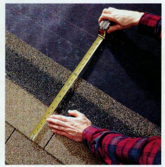
7 Check the alignment of the shingles after each 4course cycle. In several spots on the last installed course, measure from the bottom edge of a shingle to the nearest felt paper line. If you discover any misalignment, make minor adjustments over the next few rows until it's corrected.
