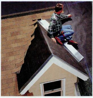
8 When you reach obstructions, such as dormers, install a full course of shingles above them so you can retain your shingle offset pattern. On the unshingled side of the obstruction, snap another vertical reference line, using the shingles above the obstruction as a guide.
