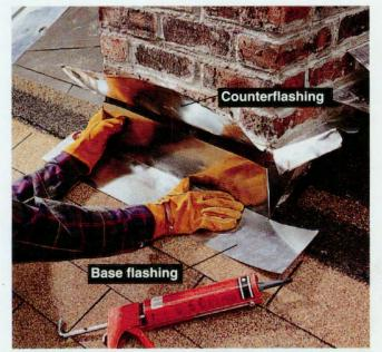
Shingle up to the chimney base. Use the old base flashing as a template to cut new flashing. Bend up the counterflashing. Apply roofing cement to the base of the chimney and the shingles just below the base. Press the base flashing into the roofing cement and bend the flashing around the edges of the chimney. Drive rubber-gasket nails through the flashing flange into the roof deck.
