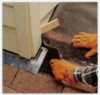
Apply roofing cement to the top side of the first piece of step flashing, where it will be covered by the next shingle course. Install the shingle by pressing it firmly into the roofing cement. Do not nail through the flashing underneath.
