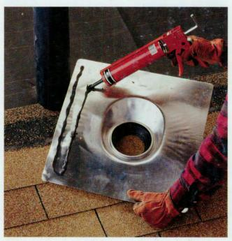
**12** Install shingles up to the vent pipe so the flashing rests on at least one row of shingles. Apply a heavy, double bead of roofing cement along the bottom edge of the flange.
