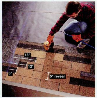
**5** Use the vertical reference line to establish a shingle pattern with slots that are offset by 6" in succeeding courses. Tack down a shingle 6" to one side of the vertical line, 5" above the bottom edge of the first-course shingles, to start the second row. Tack down shingles for the third and fourth courses, 12" and 18" from the vertical line. Butt the fifth course against the line.
