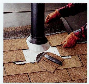
Cut shingles to fit around the neck of the flashing so they lie flat against the flange. Do not drive roofing nails through the flashing. Instead, apply roofing cement to the back of shingles where they lie over the flashing.
