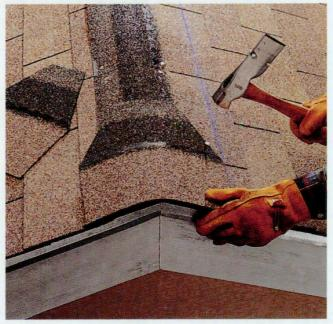
**24** Snap a chalk line 6" down from the ridge, parallel to the peak. Attach cap shingles, starting at one end of the ridge, aligned with the chalk line. Drive two 1<sup>¼</sup>" roofing nails per cap, about 1" from each edge, just below the seal strip.
