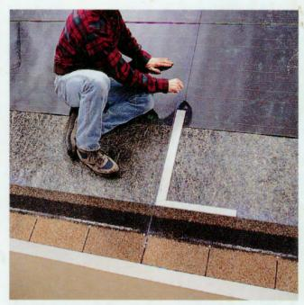
A Snap a chalk line from the eaves edge to the ridge to create a vertical line to align the shingles. Choose an area with no obstructions, as close as possible to the center of the roof. The chalk line should pass through a slot or a shingle edge on the first full shingle course. Use a carpenter's square to establish a line perpendicular to the eaves edge.
