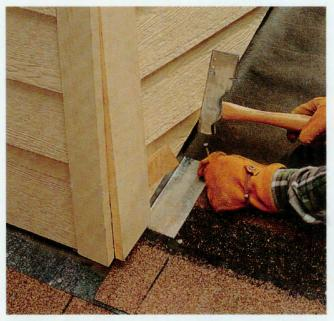
Tuck another piece of flashing under the trim or siding, overlapping the first piece of flashing at least 2". Set the flashing into roofing cement applied on the top of the shingle. Nail the shingle in place without driving nails through the flashing. Install flashing up to the top of the element the same way. Trim the last piece of flashing to fit the top corner of the element. Reattach the siding and trim.
