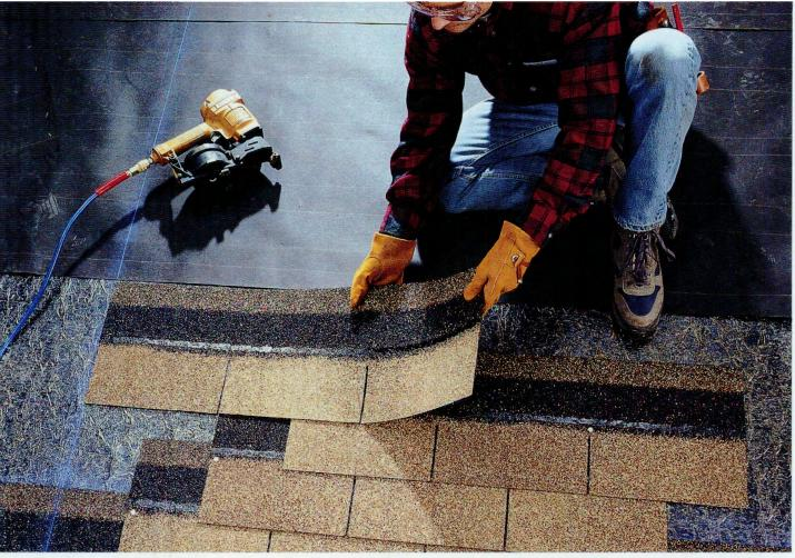
**Stagger shingles** for effective protection against leaks. If the tab slots are aligned in successive rows, water forms channels, increasing erosion of the mineral surface of the shingles. Creating a 6" offset between rows of shingles—with the 3-tab shingles shown above—ensures that the tab slots do not align.
