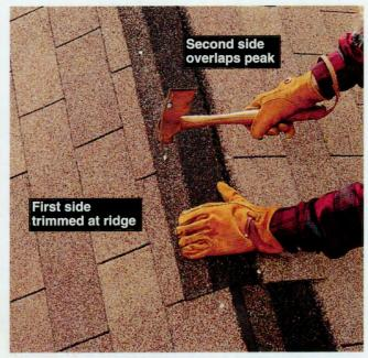
**22** When you reach a hip or ridge, shingle up the first side until the top of the uppermost reveal area is within 5" of the hip or ridge. Trim the shingles along the peak. Install shingles on the opposite side of the hip or ridge. Overlap the peak no more than 5".
