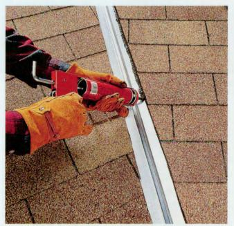
After all shingles are installed, trim them at the valleys to create a gap that's 3" wide at the top and widens at a rate of %" per foot as it moves downward. Use a utility knife and straightedge to cut the shingles, making sure not to cut through the valley flashing. At the valleys, seal the undersides and edges of shingles with roofing cement. Also cover exposed nail heads with roofing cement.
