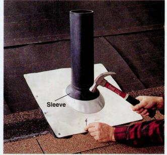
Place the flashing over the vent pipe. Position the flashing collar so the longer portion of the tapered neck slopes down the roof and the flange lies over the shingles. Nail the perimeter of the flange, using rubber-gasket nails.
