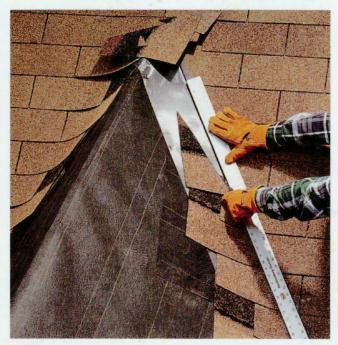
**10** Trim off excess shingle material at the V in the valley flashing, using a utility knife and straightedge. Do not cut into the flashing. The edges will be trimmed back farther at a slight taper after both roof decks are completely shingled.
