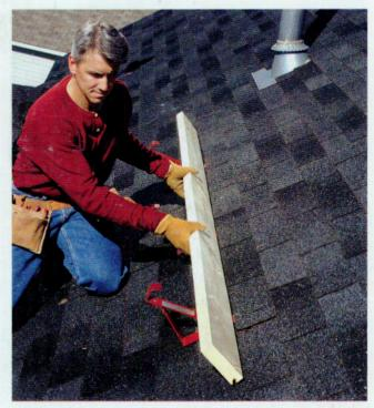
**Use roof jacks** on steep roofs. Nail the supports at the fourth or fifth course of shingles, and add the widest board the supports will hold.
