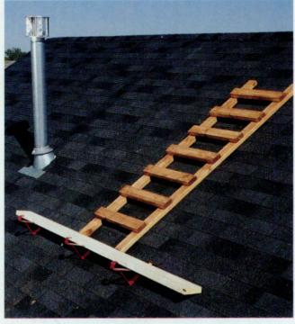
For more secure footing, fashion a roofing ladder by nailing wood strips across a pair of  $2 \times 4s$ . Secure the ladder to the roof jacks, and use it to maintain your footing.
