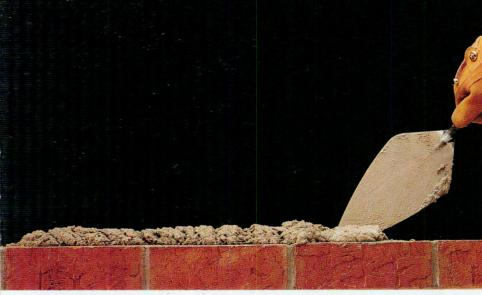
**Throwing mortar** is a quick, smooth technique that requires practice. Load the trowel with mortar, then position the trowel a few inches above the starting point. In one motion, begin turning your wrist over and quickly move the trowel across the surface to spread mortar consistently. Proper mortar-throwing results in a rounded line about  $2\frac{1}{2}$  wide and about 2 ft. long.
