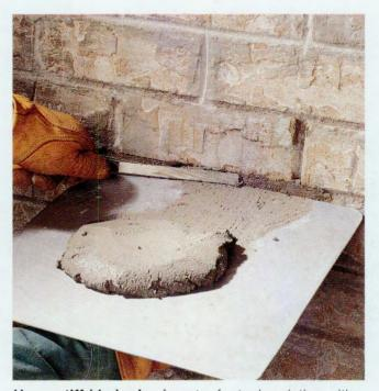
Use a stiff (dry) mix of mortar for tuck-pointing-it's less likely to shrink and crack. Start by mixing Type N mortar mix with half the recommended water. Let the mixture stand for one hour, then add the remaining water and finish mixing.
