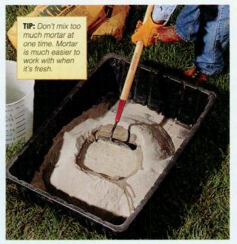
■ Empty mortar mix into a mortar box and form a depression in the center. Add about ¾ of the recommended amount of water into the depression, then mix it in with a masonry hoe. Don't overwork the mortar. Continue adding small amounts of water and mixing until the mortar reaches the proper consistency.
