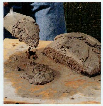
3 Snap the trowel gently downward to dislodge excess mortar clinging to the edges. Position the trowel at the starting point, and "throw" a line of mortar onto the building surface. A good amount is enough to set three bricks. Don't get ahead of yourself. If you throw too much mortar, it will set before you're ready.
