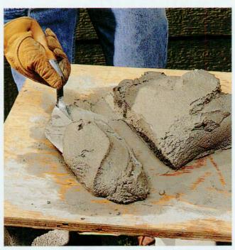
**2** Set a piece of plywood on blocks at a convenient height, and place a shovelful of mortar onto the surface. Slice off a strip of mortar from the pile, using the edge of your mason's trowel. Slip the trowel point-first under the section of mortar and lift it up.
