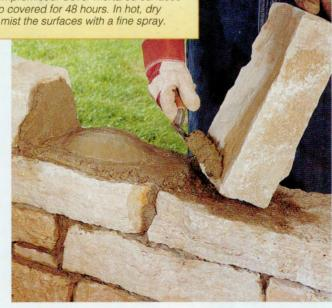
Practice buttering stones so that each buttered surface fills the gap between one stone and the next. If the mating (adjoining) surfaces are highly contoured, butter both surfaces. You can also use the trowel to create a mound (above) or a depression to conform to the shape of the adjacent stone.
