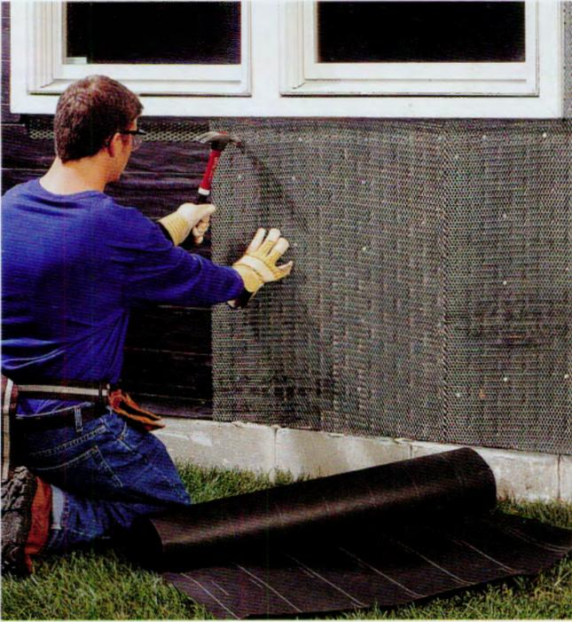
**1** Cover the wall with building paper, overlapping seams by 4". Nail or staple lath every 6" into the wall studs and midway between studs. Nails or staples should penetrate 1" into the studs. Paper and lath must extend at least 16" around corners where veneer is installed.
