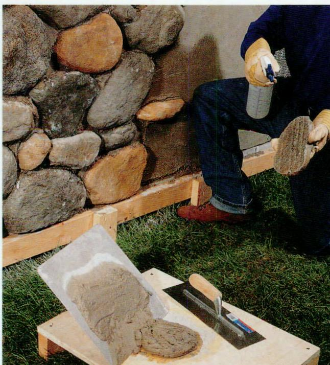
**7** Once the corner pieces are in place, install flat pieces, working from the corner toward the center of the wall.
