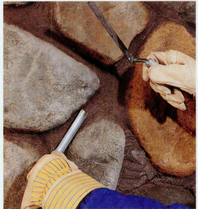
**12** Smooth the joints with a jointing tool once the mortar is firm. Once the mortar is dry to the touch, use a dry whisk broom to remove loose mortar—water or chemicals can leave permanent stains.
