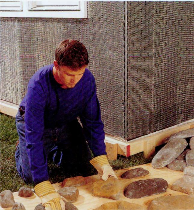
**3** Spread out the materials on the ground so you can select pieces of varying size, shape, and color, and create contrast in the overall appearance. Alternate the use of large and small, heavily textured and smooth, and thick and thin pieces.
