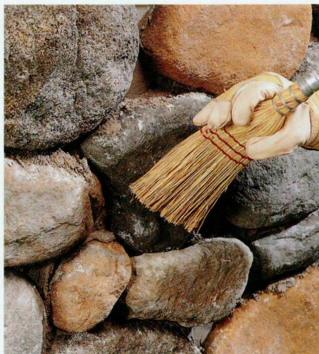
**8** If mortar becomes smeared on a stone, remove it with a whisk broom or soft-bristle brush after the mortar has begun to dry. Never use a wire brush or a wet brush of any kind.
