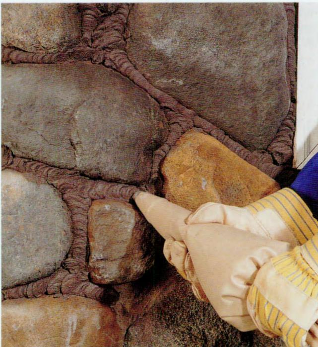
**11** Once the wall is covered in veneer, fill in the joints, using a mortar bag and tuck-pointing mortar. Take extra care to avoid smearing the mortar. You can tint the tuck-pointing mortar to complement the veneer.
