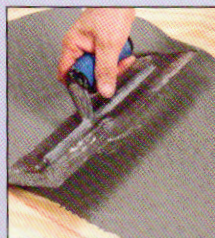
Preparing a floor for tile page 114
