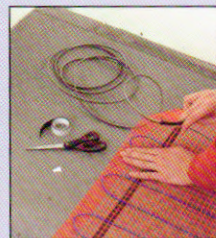
Installing electric radiant heat page 116
