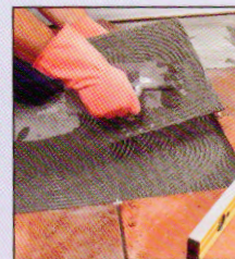
Installing ceramic floor tile page 120
